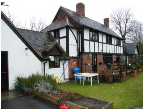
Tudor house respite centre, Brighton.
